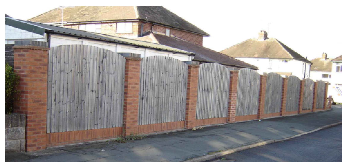
WALL WITH FENCE ABOVE
